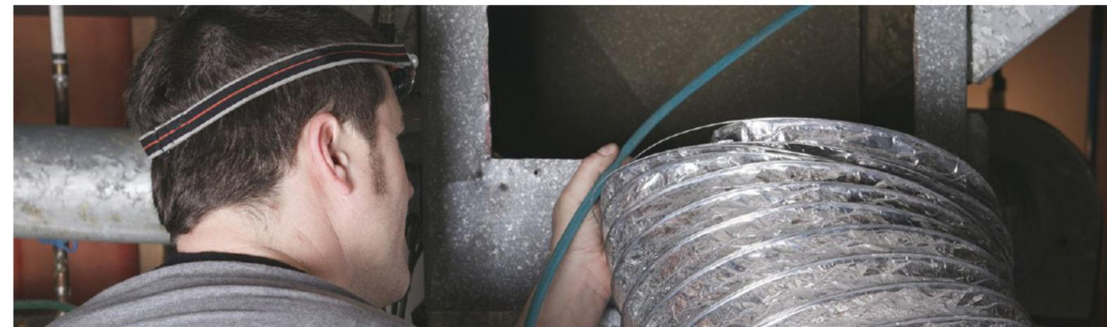
There are times when facilities managers are required to improvise when they can't obtain the correct size filters necessary for their system, and they will insert a piece of metal to close a visible gap. Although they have good intentions, this actually reduces the air flow space and creates another unnecessary problem.
